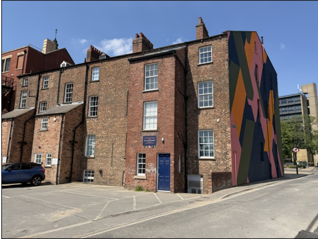
REAR CAR PARKING AREA
